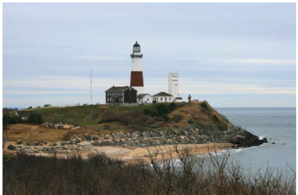
View of the Montauk Lighthouse and setting, 2007.
