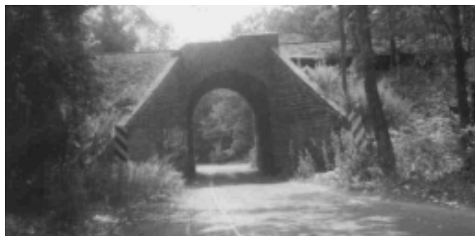
Main line Long Island Railroad bridge, East Yaphank, constructed c. 1843. CHARLA BOLTON
